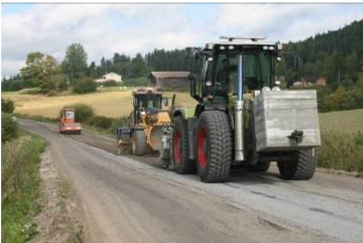
**Fig.7 MTH, grader and compacting roller**
