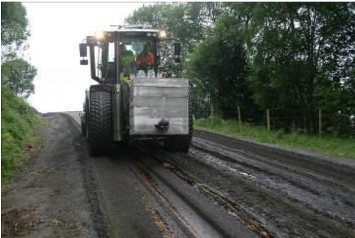
**Fig.5 Addition of lignin, in a solution of 50% dry material**
