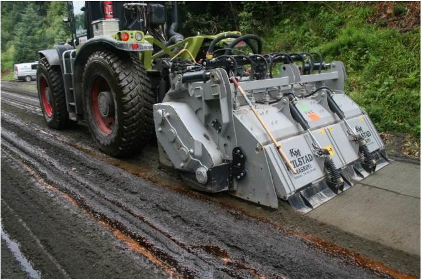
**Fig.1 MTH 225: stabilization with lignin (Norway)**
