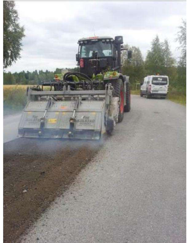
**Fig.3 and 4 Grinding the asphalt layer**
